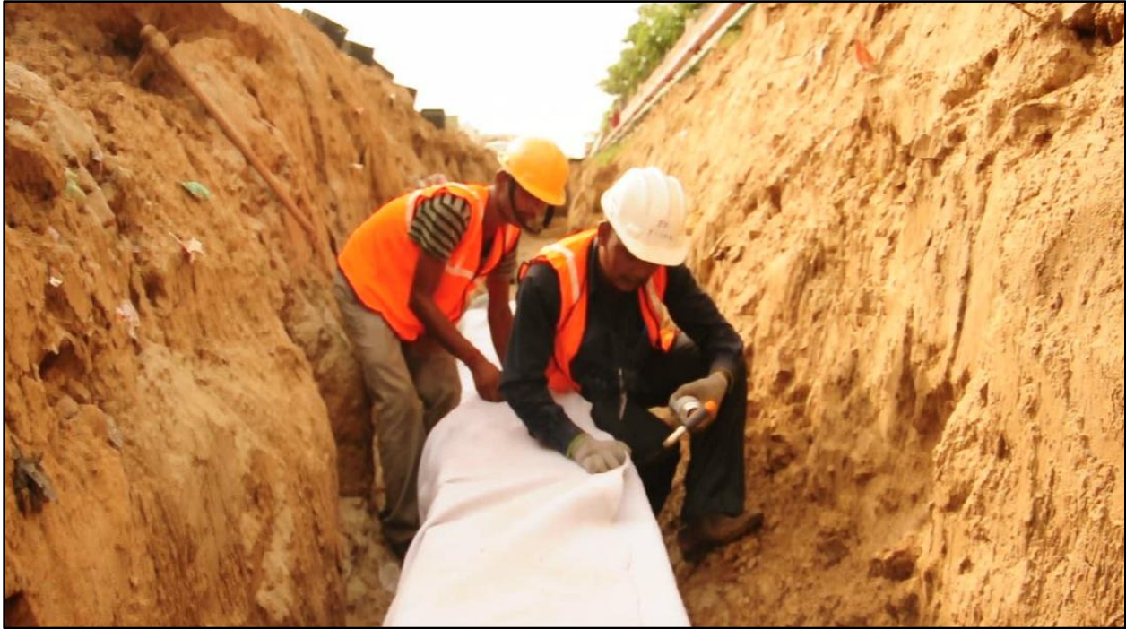
Geotextile wrapping of LifeRain™ Modules
