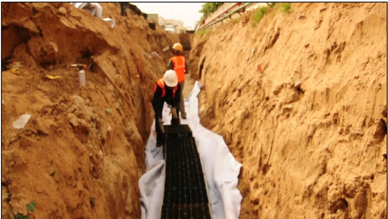
LifeRain™ Module Installation
