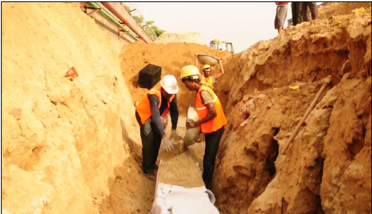
Backfilling Process
