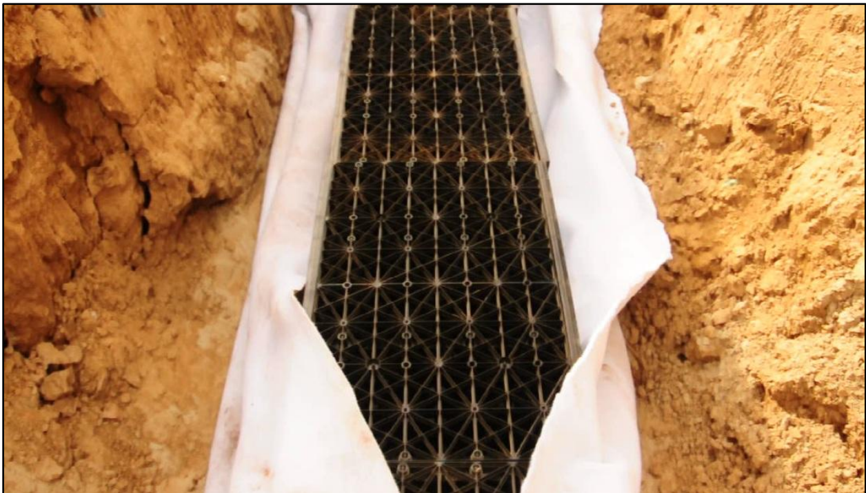
Geotextile wrapping of LifeRain™ Modules
