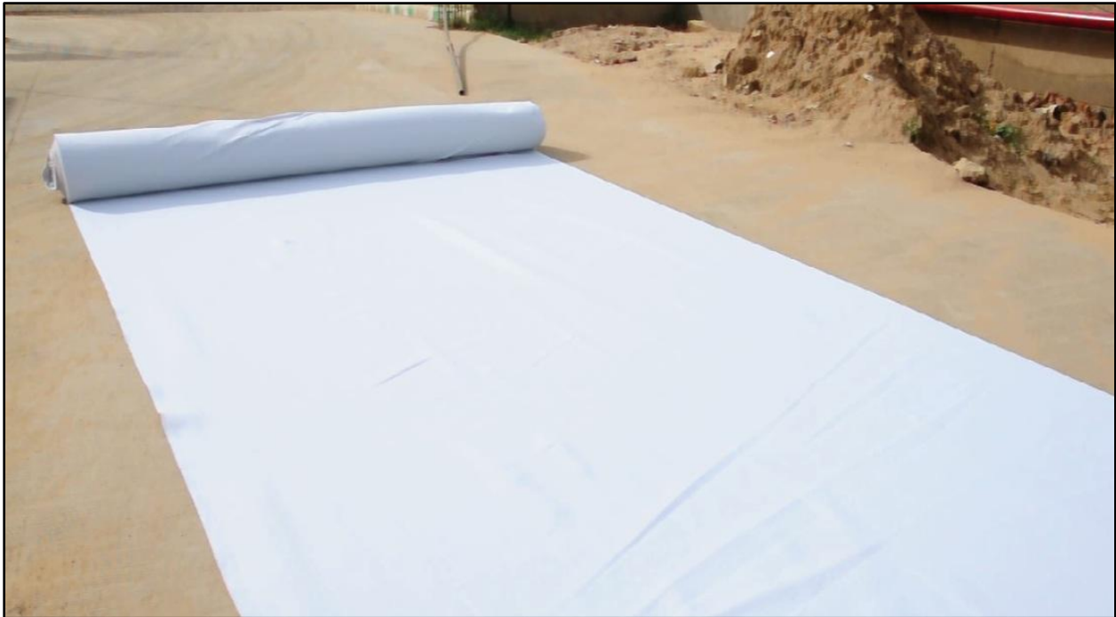
Cutting & Laying of Geotextile
