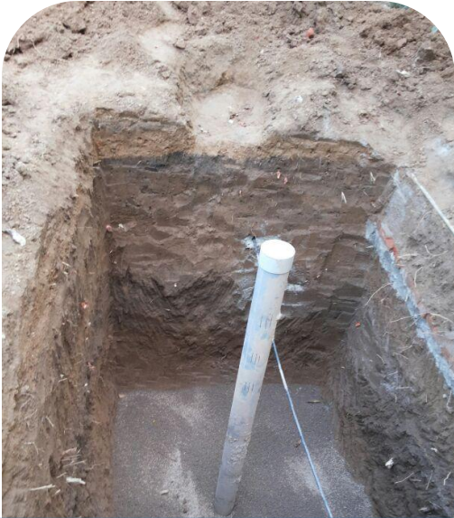
Recharge well & Base Preparation
