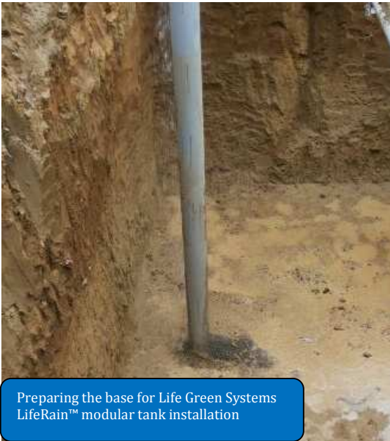
Installation of Borewell to recharge the ground water
