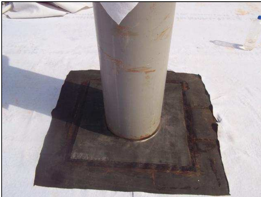
6. Observation well for extraction of water from tank
