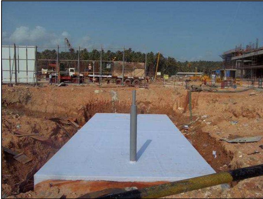
5. LifeRain™ Modules are wrapped in geotextile
