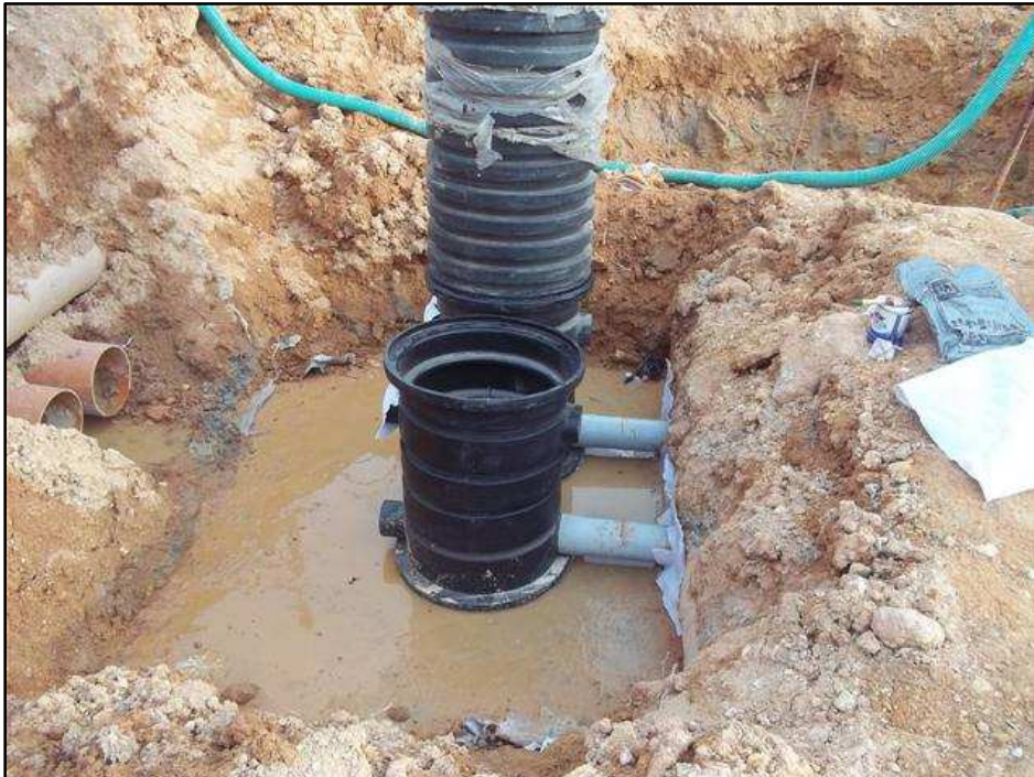
4. Installation of 4 micro filters
