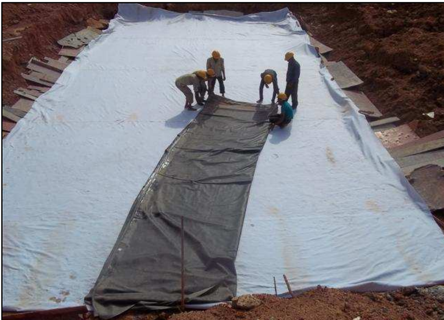
2. Laying of geotextile & EPDM liner
