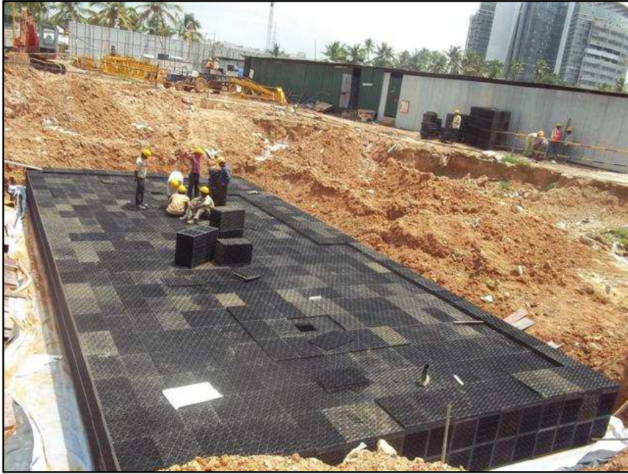
3. Assembling of LifeRain™ Modules
